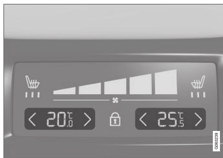
Temperature control on the climate panel at the rear of the tunnel console.
